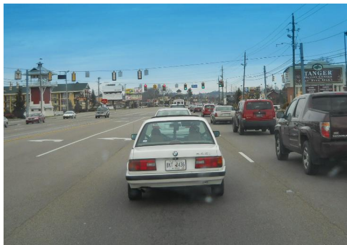
Existing traffic signal system in Sevierville
